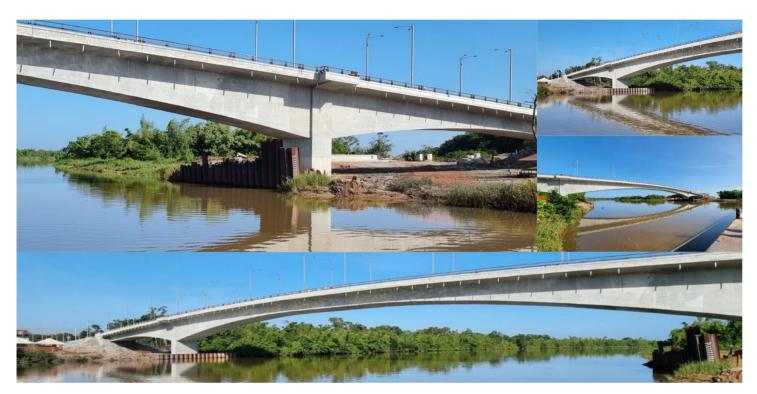
The new bridge over Wawa river, placed close to the town of Puerto Cabezas (Nicaragua), has a total length of 255m divided in three spans of 57.5+140+57.5m. It has a total width of 15.3m, allowing to accommodate a two-lanes roadway with pedestrian walkways on each side.
